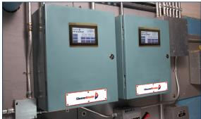
The HMI provides the operator access to the control screen, alarm history screen, and monitor I/O screen. Secured screens are provided for loop tuning and for initial system setup.
